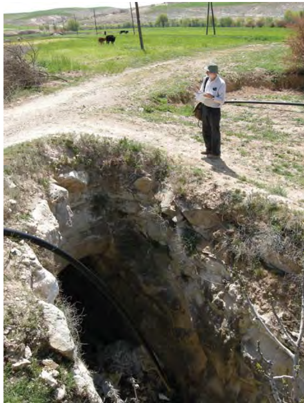
Fig. 6: Water-supply channel and tunnel cut in limestone along the north bank of the Sajur River near Tell Sha'ir South. This is probably a Roman / Byzantine channel that was re-excavated in the Late Ottoman –early modern period.
