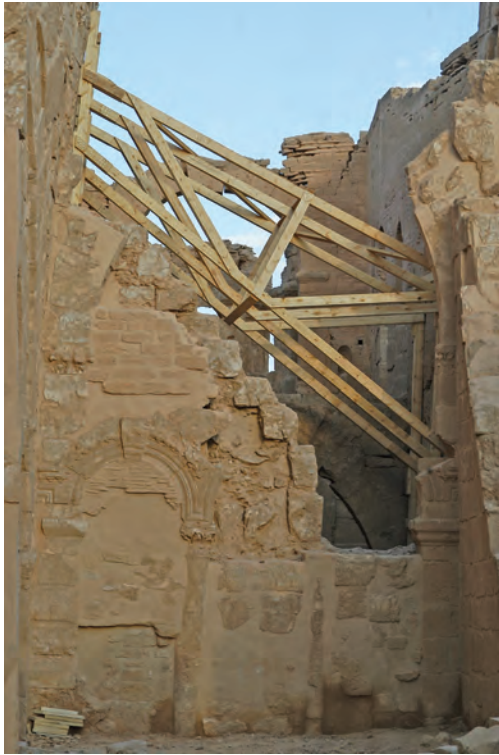
Fig. 12: Basilica A, temporary supportive construction in the south side aisle, Tobias Horn 2008.
