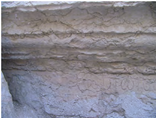
Fig. 35: Inscription of inside a well on the south side foundation of No.129-b (from the south).
