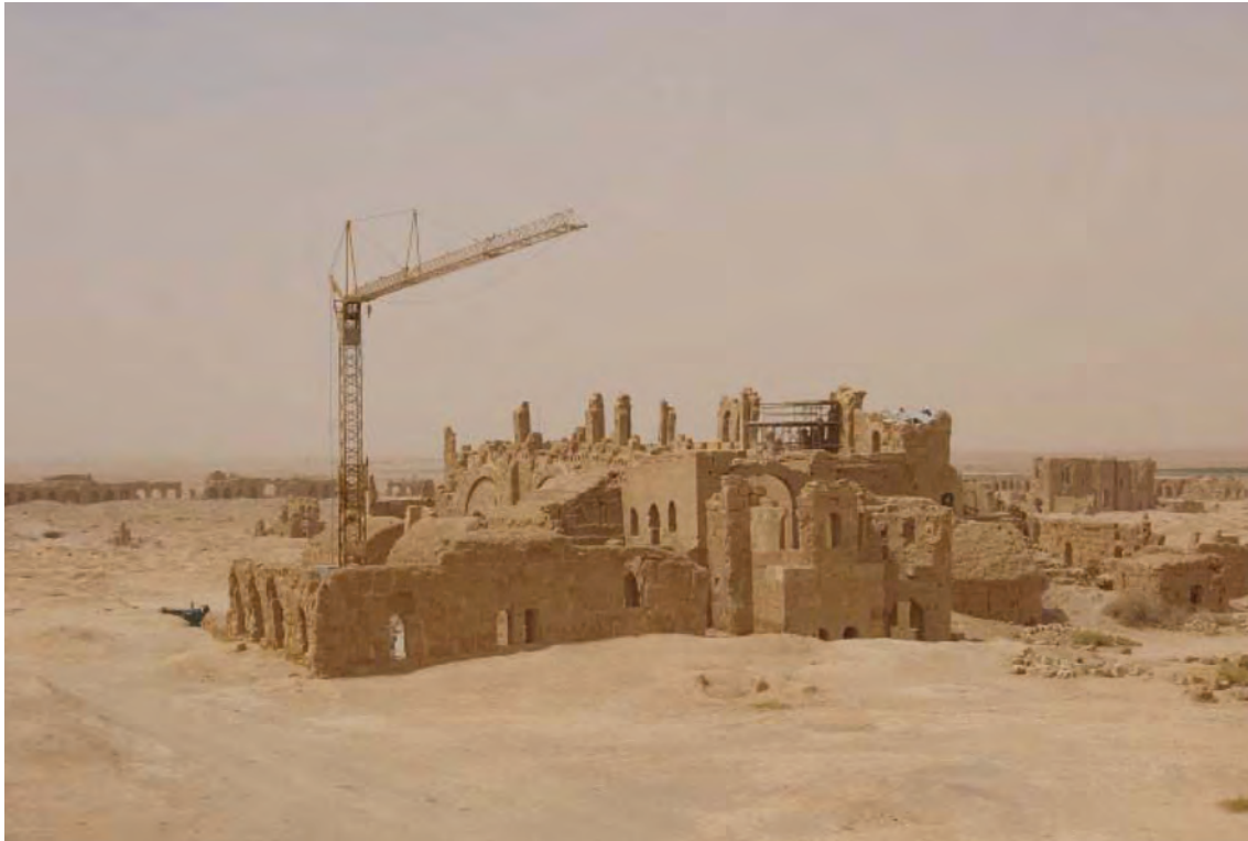
Fig.6: Resafa, Basilica A, Consolidation work, view from southeast (M. Gussone 2009).
