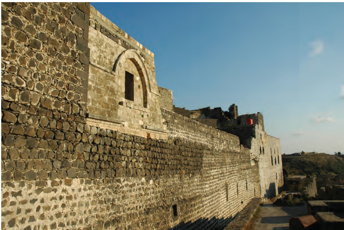
Fig. 3: The western façade of the second Chapter House with in situ window. (B. Major).
