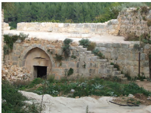
Outside view of the location of the sondage VI
