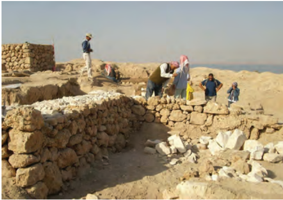
Fig. 5: Emar, temple of Ba'al, reconstruction of the retaining wall in the southeast.
