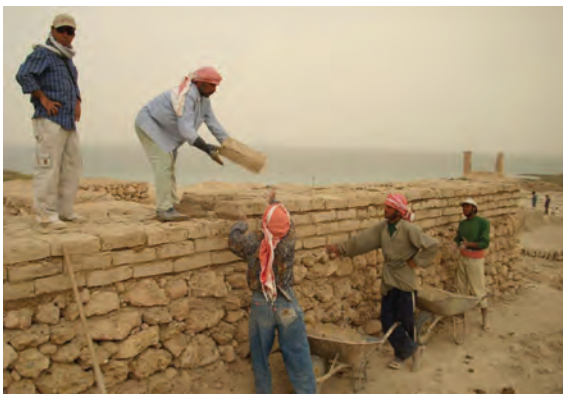
Fig. 7: Emar, south wall of the temple of Ba'al. Bonding mud bricks.
