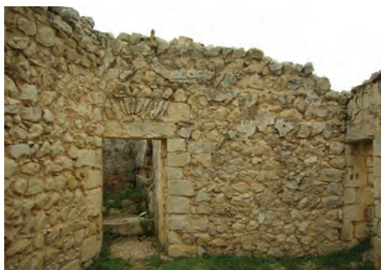
Orthophotograph of an inner wall of the Mamluk bath
