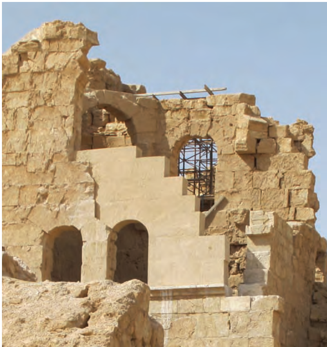
Fig. 7: Basilica A, relic chapel, east wall, due to structural reasons part of the collapsed wall had to be reconstructed (T. Horn, 2010).
