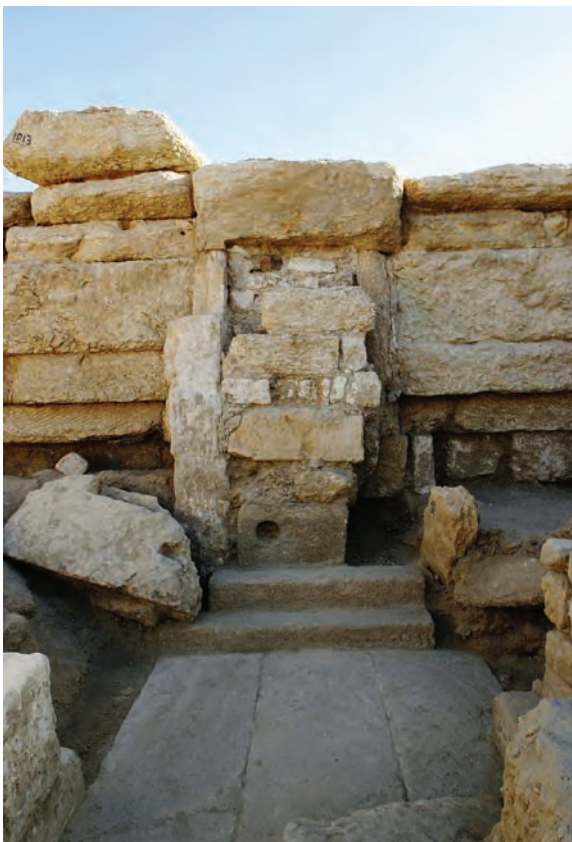
Fig. 16: A gate and a stairs attached to the south side foundation (from the inside).
